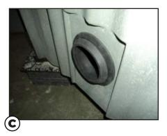
(4) Install rubber grommet, make sure the larger tapered flange goes into hole in blind
