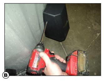
(8) Secure snorkel to outlet tube using two screws
